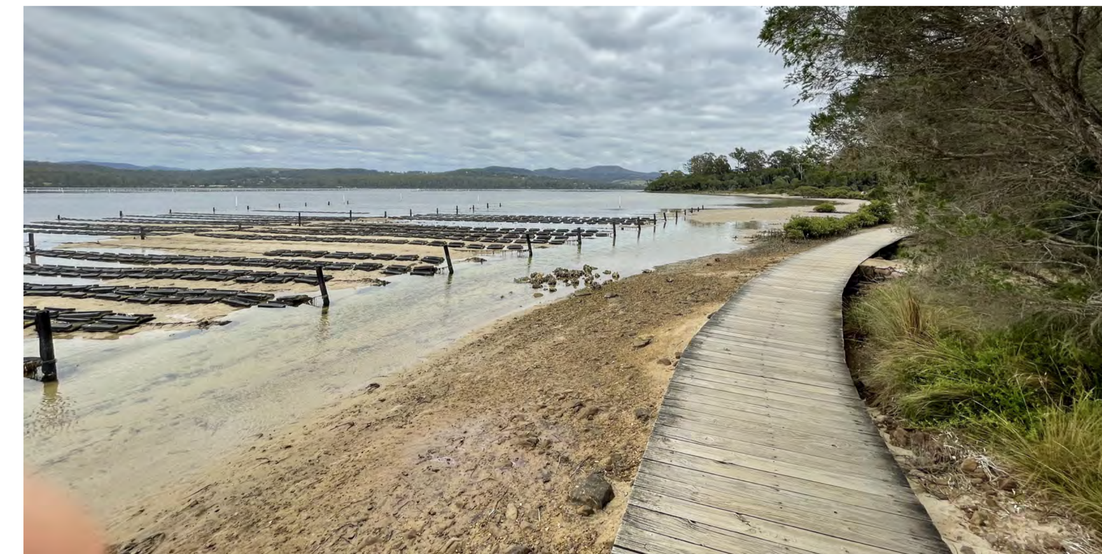
The curved alignment is attractive, however all timber decking has a limited lifespan. This alignment is maintained for the more rational geometry required by FRP deck panels.
