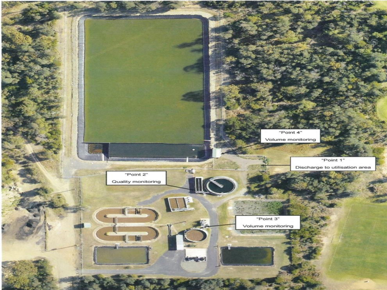
8, 9 MAP – TATHRA SEWAGE TREATMENT PLANT
