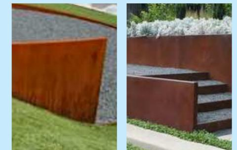
Corten steel blade retaining wall examples
